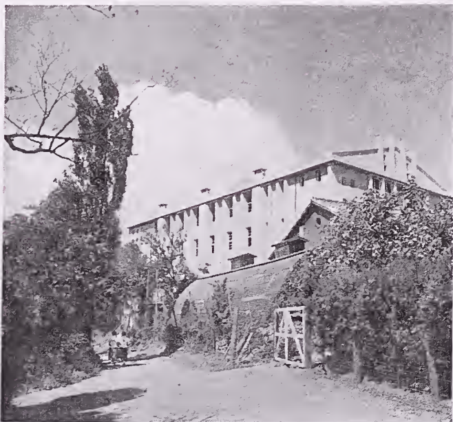
Sinmyung girls' school building was completed just last year with aid of Presbyterian Women's Organizations. It is for middle grades and high school. It houses 1,200 students.
